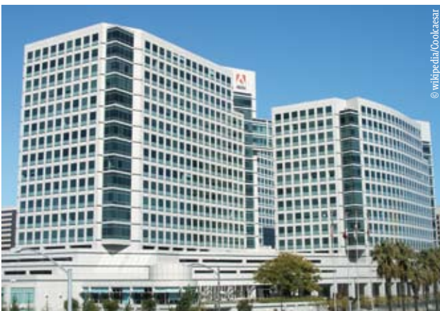
Adobe invested $1.4M to improve the energy efficiency of their San Jose headquarters
